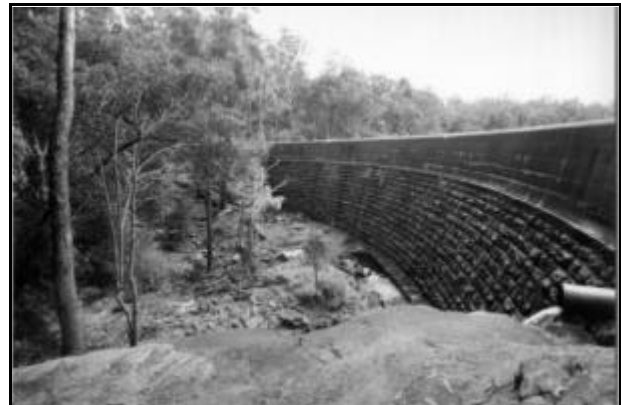
Lake Parramatta dam wall
