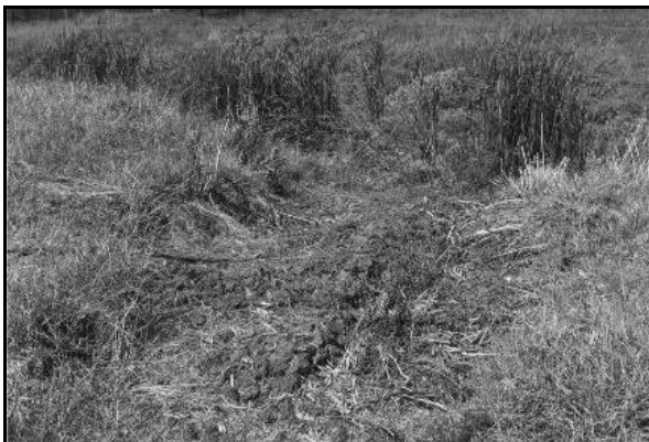
Bank stabilisation at Blacktown Creek (above)
