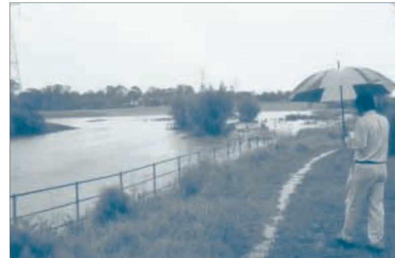
McCoy Park flood retarding basin was built on Toongabbie Creek at Toongabbie to temporarily contain flood waters such as during the January 2000 flood.
