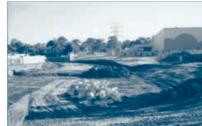
Construction of the Myrtle Street-Ollier Crescent flood retarding basin at Prospect.
