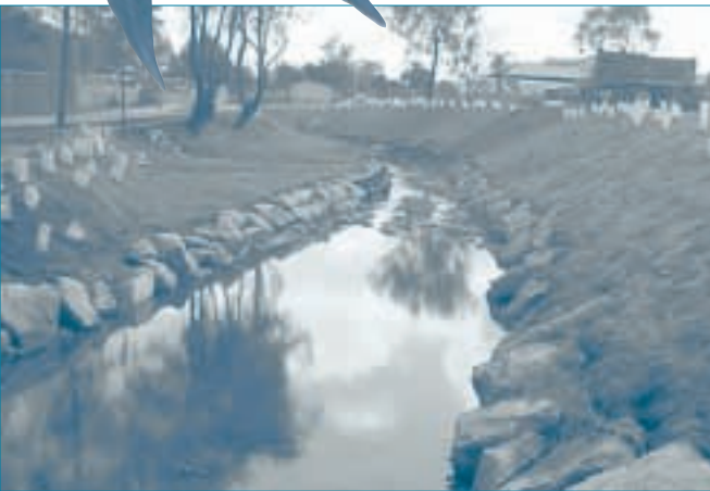
Greystanes Creek reconstruction adjacent to Toongabbie Bowling Club, Toongabbie.
