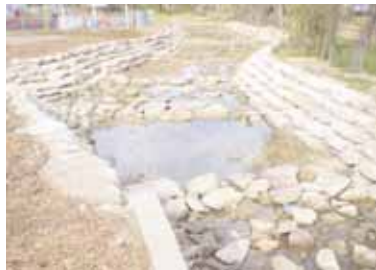
Pendle Hill Creek Floodway
