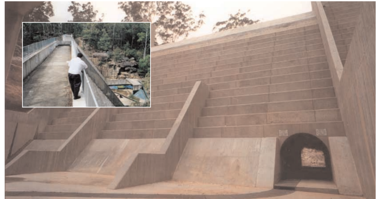
The Basin is formed by a 30 metre high by 110 metre long concrete wall and associated structures, including a large culvert through the base of the wall that carries dry weather flow and allows bushwalkers to pass beneath the wall. James Henderson (insert) the Trust's Stormwater Inspector undertakes regular inspections of the Basin to ensure that there are no changes in the structure which might affect its flood mitigation performance or safety
