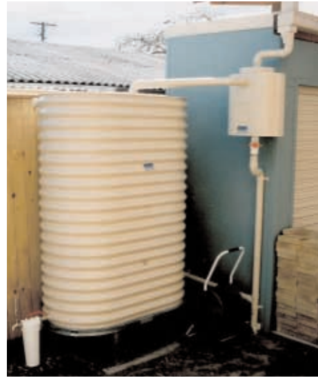
Private rainwater tanks, like this, are used as part of the Water Sensitive Urban Design process
