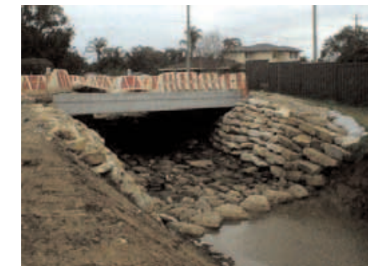
Caption: New bridge recently completed over Grantham Creek in Seven Hills
