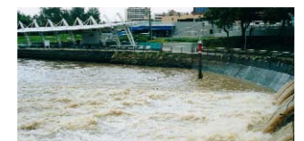
Charles Street Wharf in flood.
